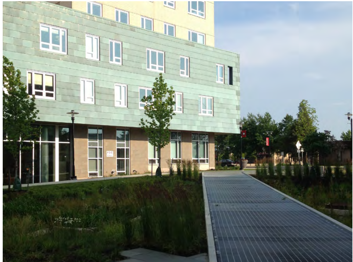
Bioswales were included in the Livingston Apartments landscape as a stormwater management strategy
