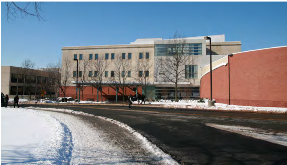
Existing view of Allison Road Classroom Building and bus stop
