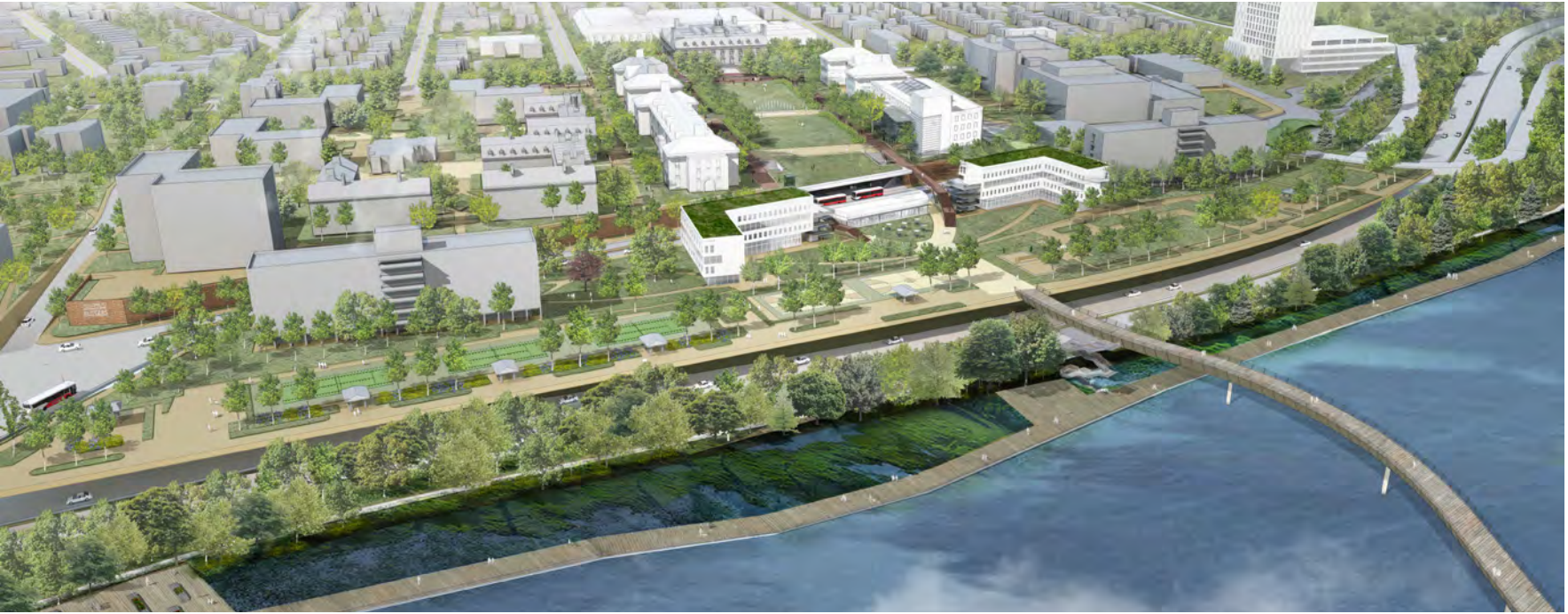
Figure 1.5: New bridge across the Raritan
